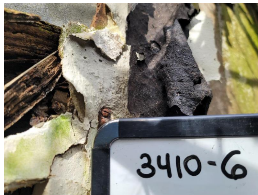
3410-6 Roof Felt Typical Exterior Roof
