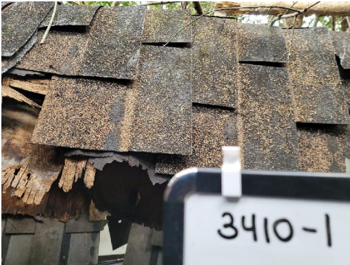
3410-1 Asphalt Shingle/Tar Typical Exterior Roof
