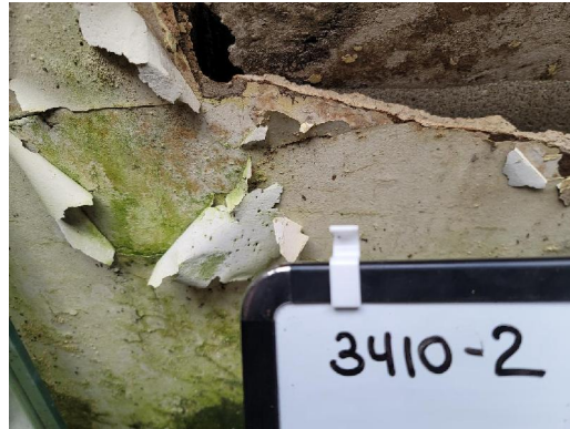
3410-2 Drywall Joint Compound/Beige (2% Chrysotile) Typical Interior Walls/Ceilings
